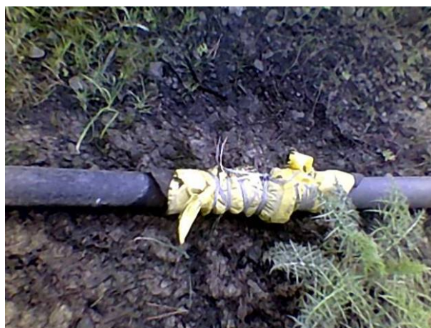
Figure 35 – Liquid waste leakage during its transfer to the evaporation pond
